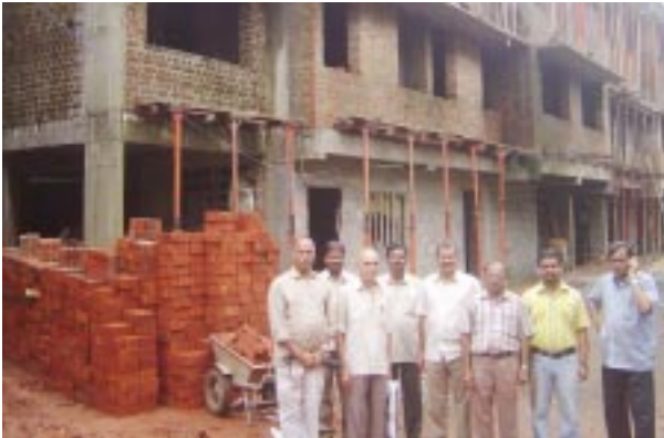
Anugraha Committee Members and Architects during the site visit
